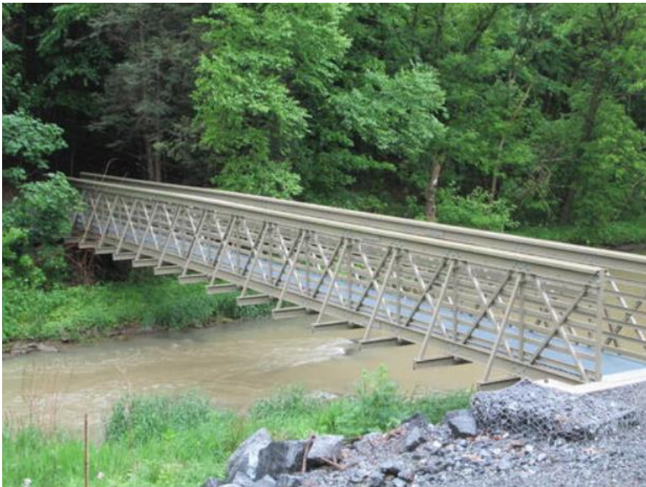
Figure 4: FRP Bridge example
